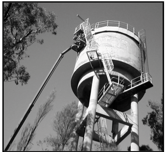
New access ladders and platforms installed by Riverina Water staff at Milbrulong Reservoir (above) and Boree Creek Reservoir (right)
