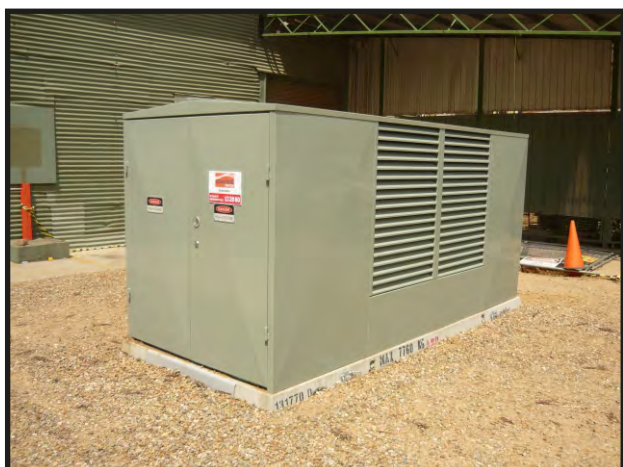
New 1500 kVA substation
