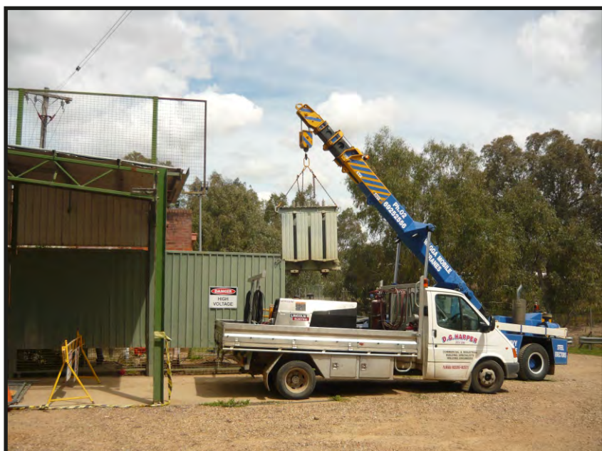
Removal of one of four old transformers
