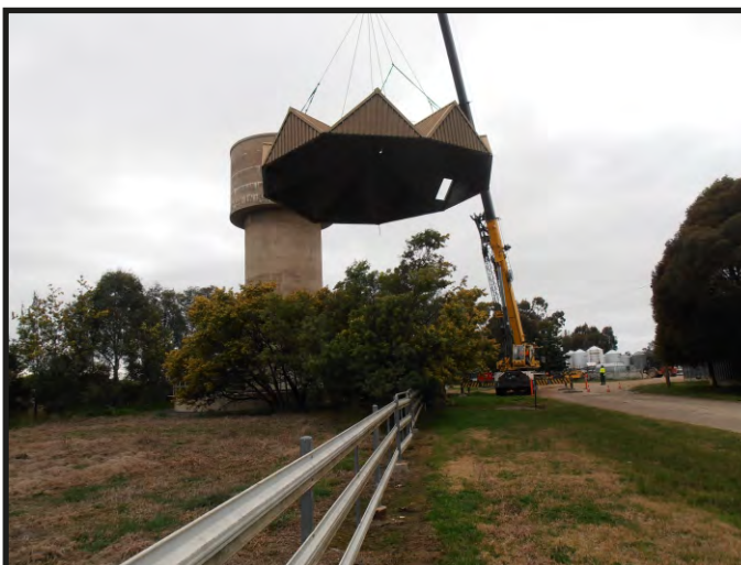
Old roof being lowered to the ground.
