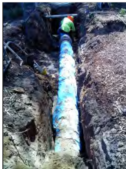
Shows the pipe being laid to make the final connection to the existing main in Morgan Street.
