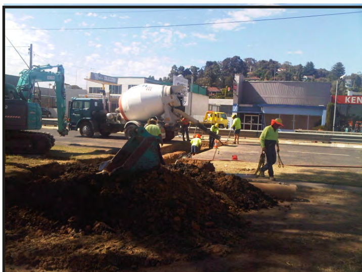
The gang making the connection in Edward St and pouring the thrust block.
