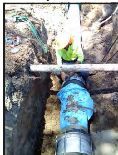
A gibault pipe connector and tapping band being fitted for connection to the irrigation system
