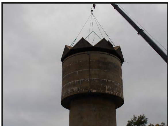
Removal of the old Crown roof
