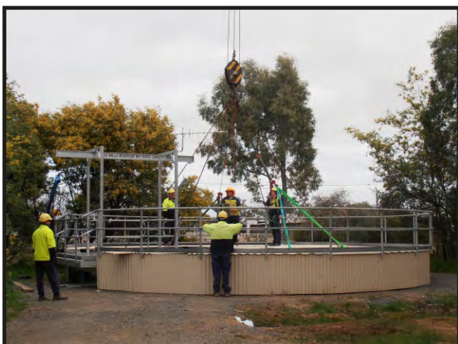
New roof was built on the ground
