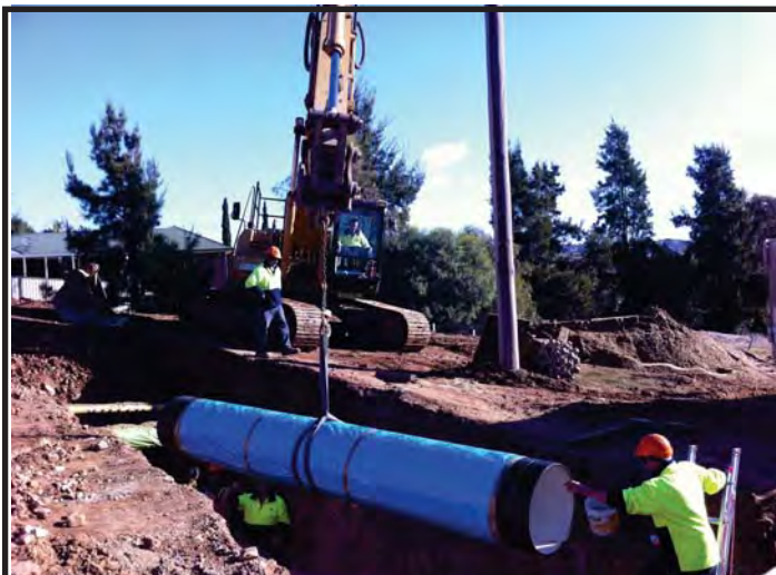
Pipeline Construction under Red Hill Road by Riverina Water staff
