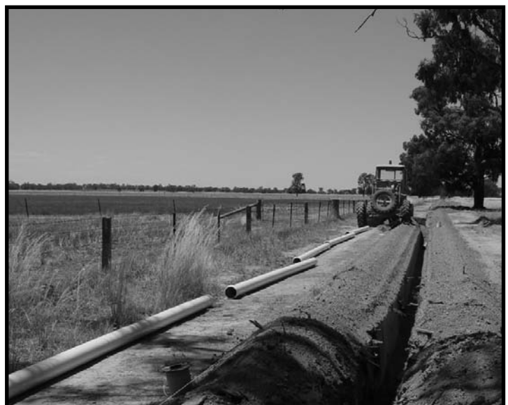
21.7km of 150mm OPVC Class 12 Vinidex pipe laid by Riverina Water staff
