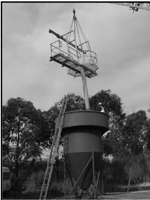
Setting up Tarcutta Candy Tanks For Treatment Trials June 2005
