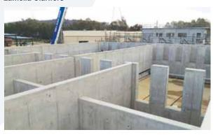
The Lamella Clarifiers will remove most of the solids from the river water before filtration. The photo shows the completed concrete tanks following successful hydrostatic (leak) testing.
