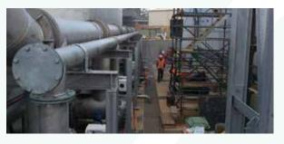
The photo shows the pipe gallery. The pipes collect water from the filters before being transferred to the filtered water tank
