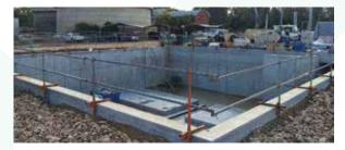
The clear water storage tank is the last part of the water treatment process before the water is pumped into the distribution system. This photo shows the completed tank with concrete panels on the floor. The panels will be erected in the tank as baffles to provide a chanel flow path for chlorine disinfection.
