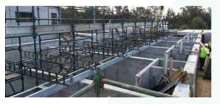
The filters will contain anthracite coal, sand, and garnet to remove remaining solids from the water. This photo shows the completed concrete cells with scaffolding installed to allow construction of internal components
