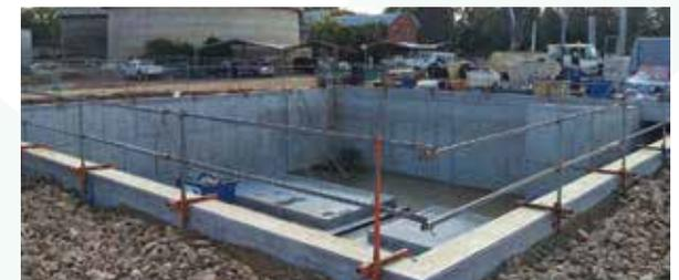
The clear water storage tank is the last part of the water treatment process before the water is pumped into the distribution system. This photo shows the completed tank with concrete panels on the floor. The panels will be erected in the tank as baffles to provide a channel flow path for chlorine disinfection.
