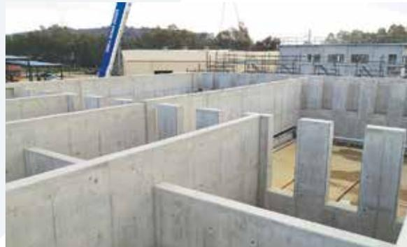
The Lamella Clarifiers will remove most of the solids from the river water before filtration. The photo shows the completed concrete tanks following successful hydrostatic (leak) testing.
