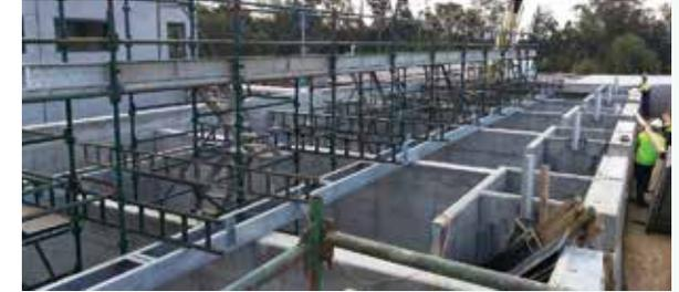
The filters will contain anthracite coal, sand, and garnet to remove remaining solids from the water. This photo shows the completed concrete cells with scaffolding installed to allow construction of internal components
