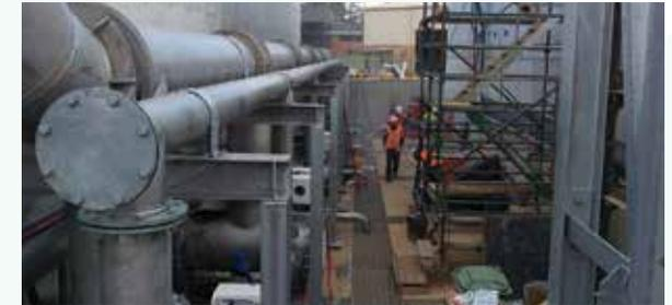
The photo shows the pipe gallery. The pipes collect water from the filters before being transferred to the filtered water tank
