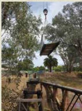
*This photo is of the old footbridge being removed as the bridge decking was old and worn. The old timber support piles have been replaced by new steel piles.*
